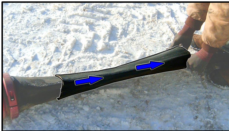
Figure 15 - Pull Repair Sleeve
